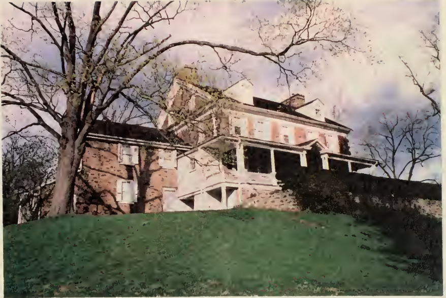
Figure 7. Mill Grove mansion, existing appearance of south and west elevations showing the addition of later details to the original plan. (1994)
